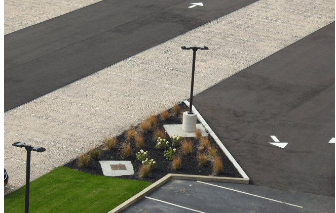
Permeable paver parking lot designed to aid in stormwater management adjacent to the boardwalk in Far Rockaway, NY.
